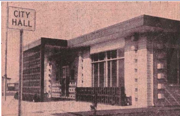
Grover Beach City Hall—154 South 8th Street
