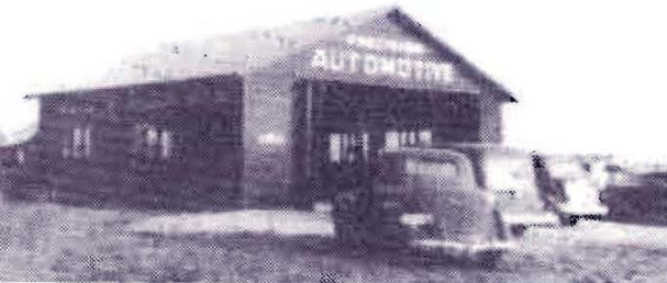
Grover Beach Fire Station—701 Rockaway Avenue "PRECISION AUTOMOTIVE"
