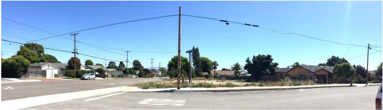
View of Site from the North
